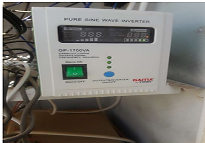
Fig. 14. AC/DC inverter (1700VA \approx 1000W).
