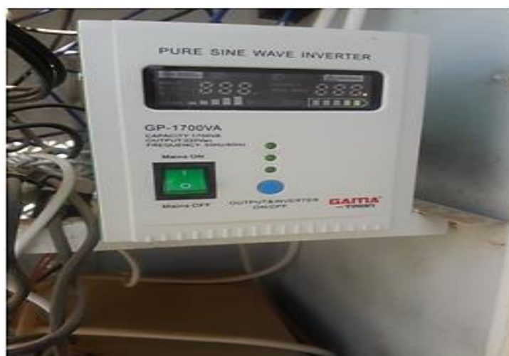
Fig. 14. AC/DC inverter (1700VA \approx 1000W).
