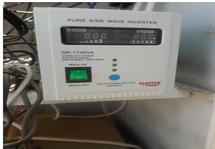
Fig. 14. AC/DC inverter (1700VA \approx 1000W).
