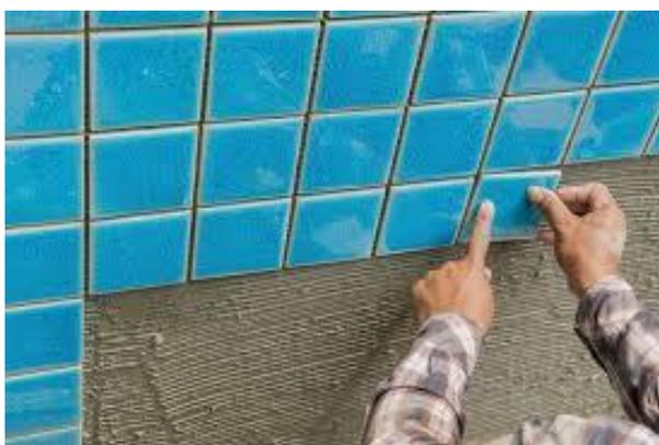
Figure (3): Installing tiles on the walls
