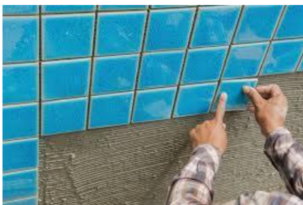
Figure (3): Installing tiles on the walls
